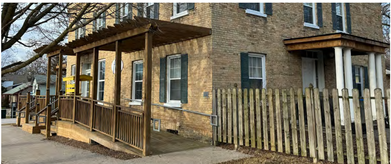
Fig.31: Example of entrance ramp attached with the least amount of damage to the building and aesthetically complementing the building (10 Bayfield Main Street North).
