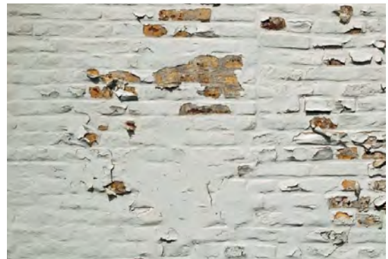
Fig.27: When painting over bricks moisture can be trapped in the wall, causing damage.
