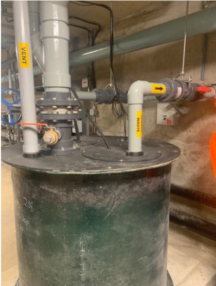
Figure 9: Sewage Ejector System
