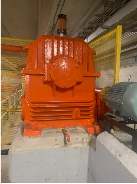
Figures 8a and 8b: Flocculation gear drives
