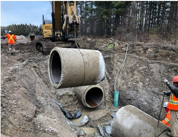
Figure 5a: Removal of pipe #4-80
