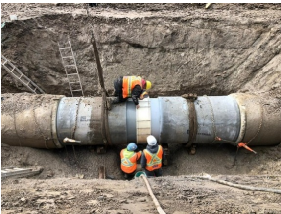
Figure 5c: Installation of dresser coupling
