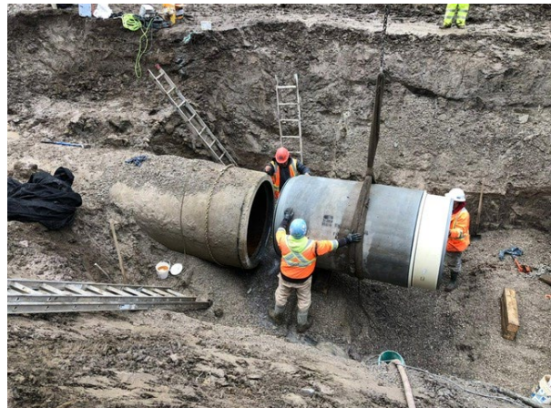
Figure 5b: Installation of repair piece
