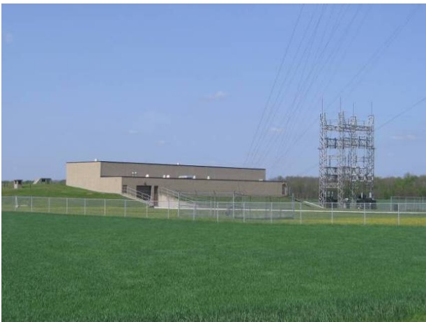
Figure 1: McGillivray Booster Pumping Station
