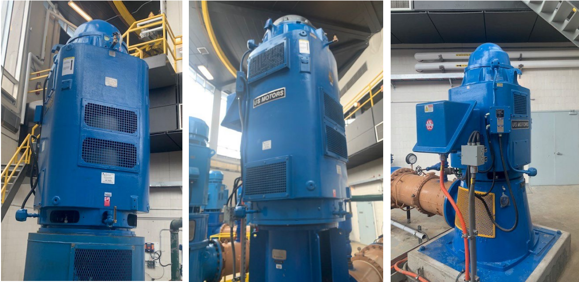
Figures 7a, 7b, 7c: Low lift motors #2, #5 and #6
