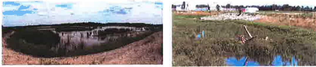
Figure 13 - Sludge Containment Wetlands
